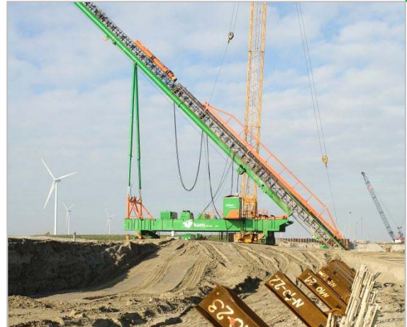
Kademuren Wilhelminahaven, Eemshaven
