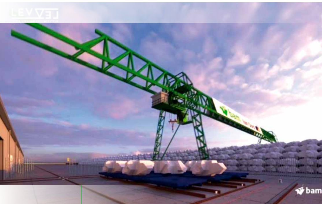
The Xbloc factory in Harlingen is constructed in a circular way. When the construction of the Afsluitdijk is finished, the factory is dismantled to be used elsewhere
