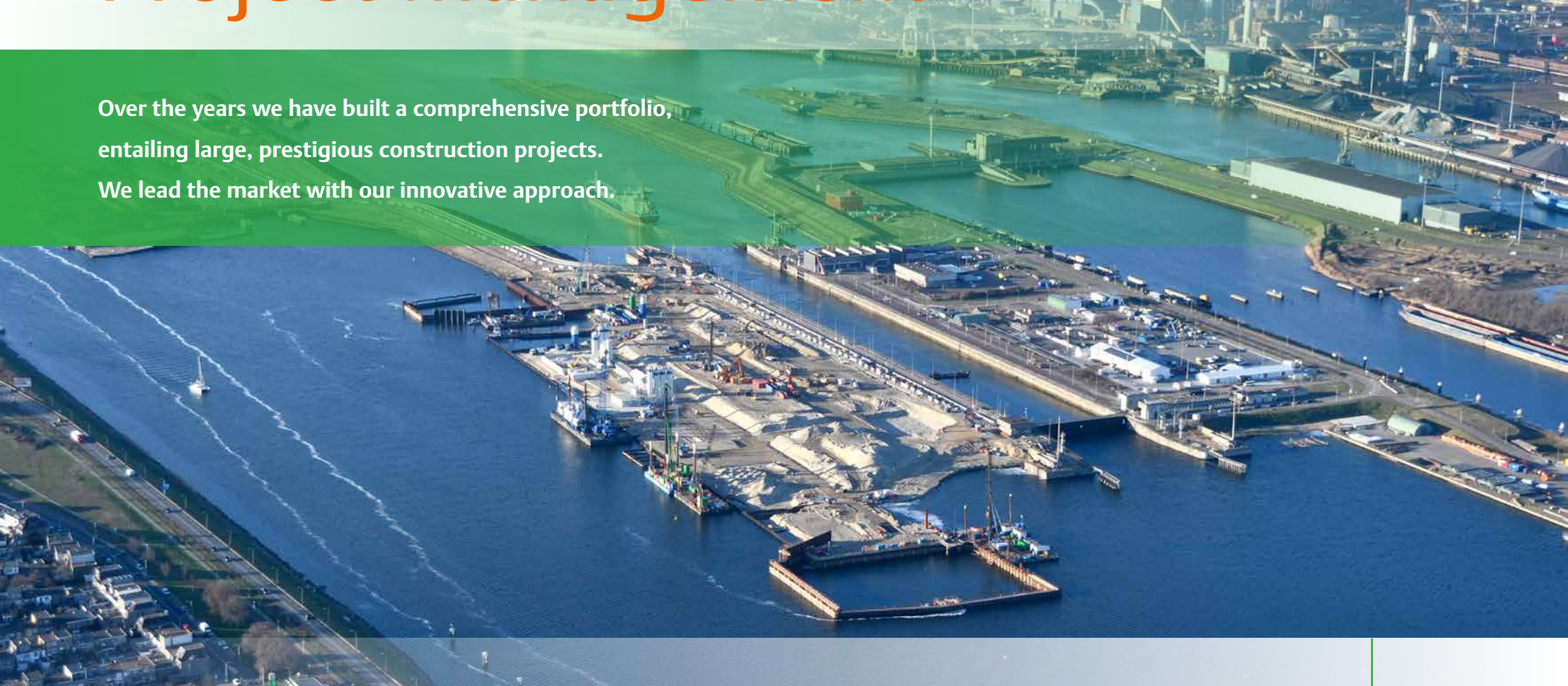
Sea Lock IJmuiden during construction
