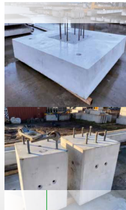
Photos of a modular foundation of a TenneT land station
