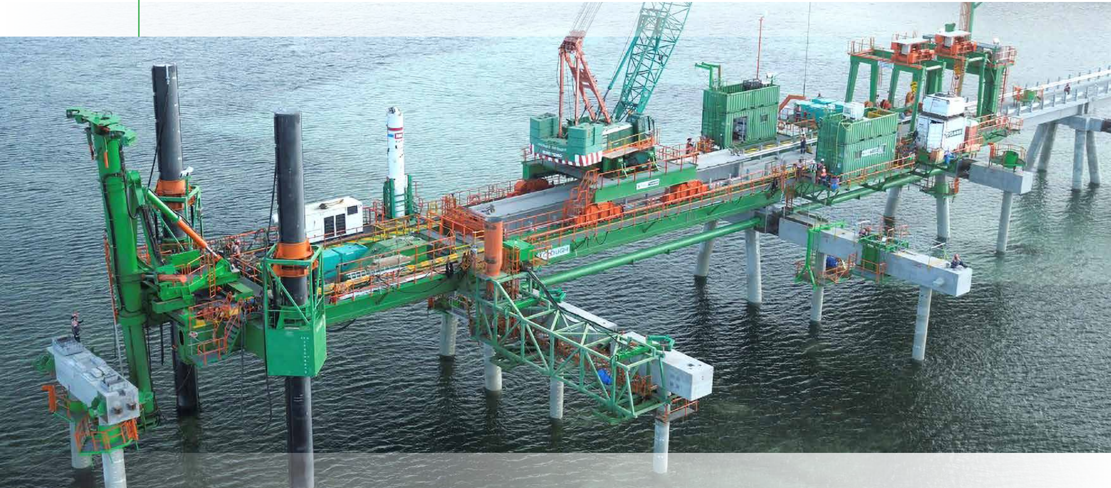
LNG jetty built by BAM and partners
