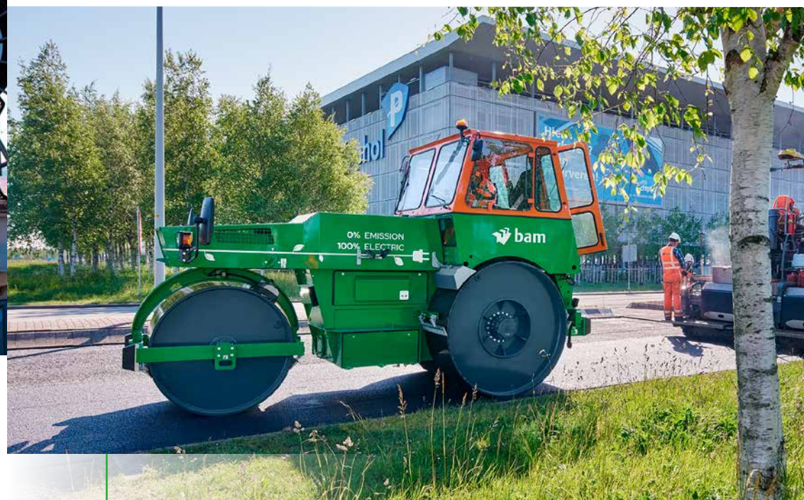
World's first electric asphalt roller by BAM Infra
