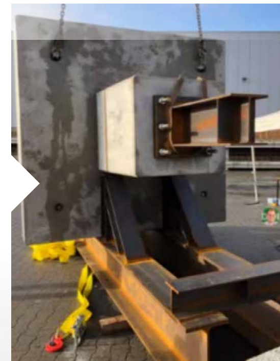
Photos of a modular foundation of a TenneT land station
